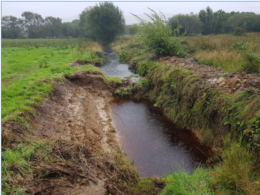
Figure 3 In-ditch wetland under construction. Note reprofiled drain with shelves of different depths creating different depths and widening the drain. Earth bunds are also visible as barrier to slow the flow of water within the drain. (source: Pearl Mussel Project)
