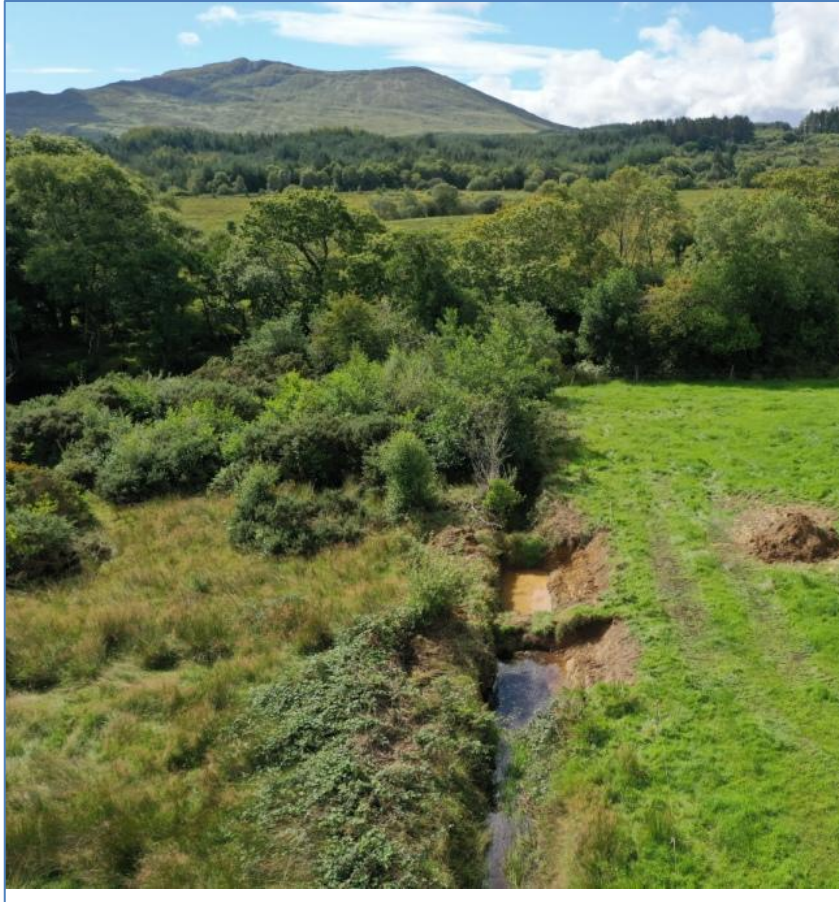
Figure 4 Note widened sections of the drain. There are usually two widened chambers connected by a dam with pipe to allow water to flow through. (source: Pearl Mussel Project)
